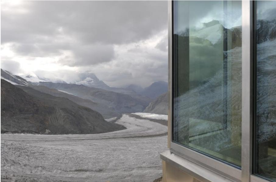
The insulated glass panes of the new Monte Rosa Hut are characterized by a combination of solar and thermal protection. The COMBI glass panes not only provide for effective basic solar protection but also create a cosy atmosphere inside the room by maintaining a low heat loss.
