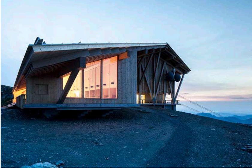
The Chäserrugg mountain restaurant 2,262 metres above sea level in the canton of St. Gallen makes an impressive sight thanks to the successful combination of traditional timber construction and large glass elements. As a result of the low  $U_g$  value, the triple insulation glazing with SILVERSTAR ZERO Eplus thermal insulation coating maintains a pleasant room climate. (Photo: Juergen Pollak)
