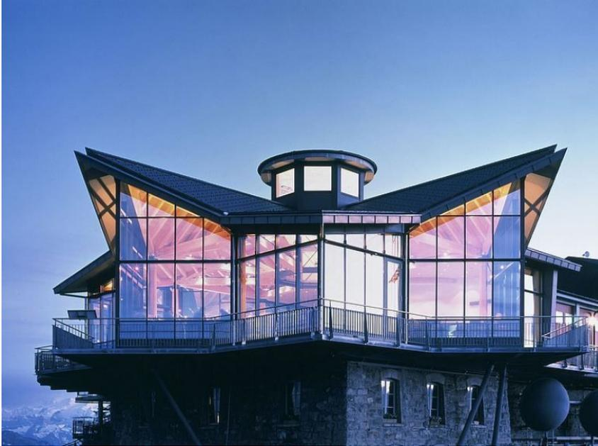
The Rondorama restaurant on the Stanserhorn is located 1,900 metres above sea level and is exposed to extreme sunlight through the large glass façade areas. Here, the solar protection glass SILVERSTAR SUNSTOP Neutral 50 T prevents the rooms from overheating.
